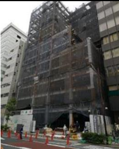
Fig 33: Hotel Vista Tokyo Tsukiji (Under Construction)
