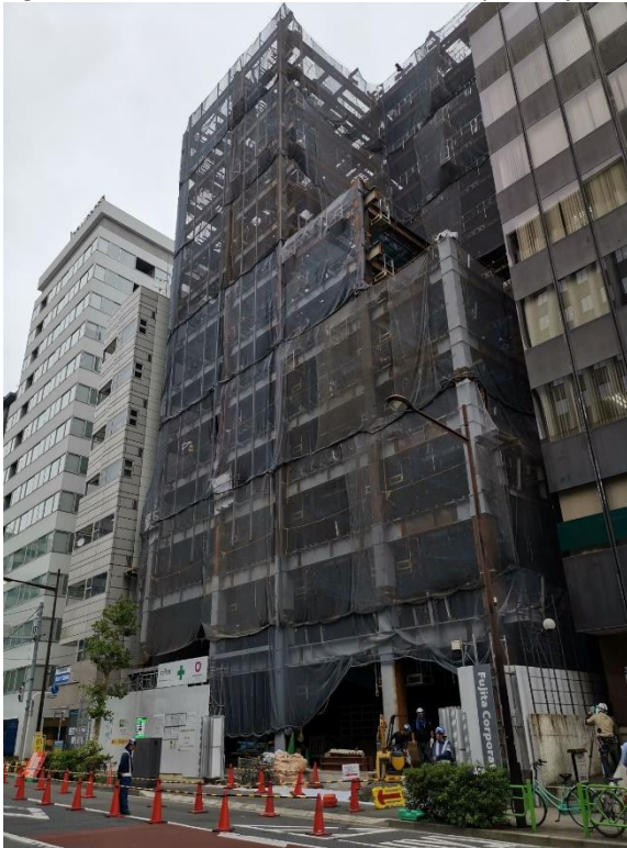
Figure 1: Construction site of Hotel Vista Tokyo Tsukiji
