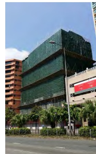
Existing building currently undergoing demolition
