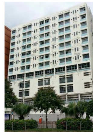
Existing building on the land before demolition
