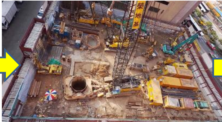
Site after demolition undergoing foundation work
