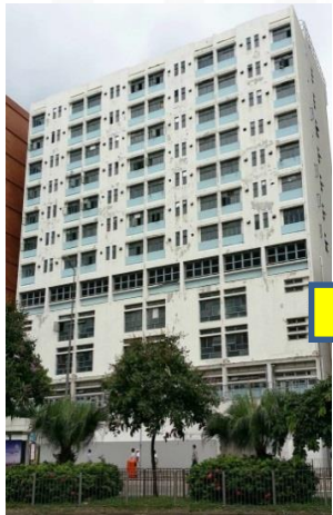
Original building on the land before demolition
