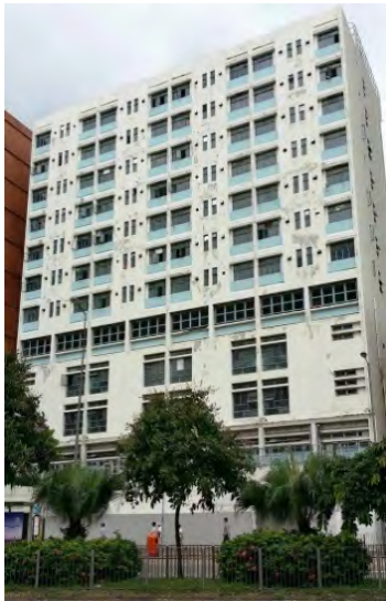
Original building on the land before demolition
