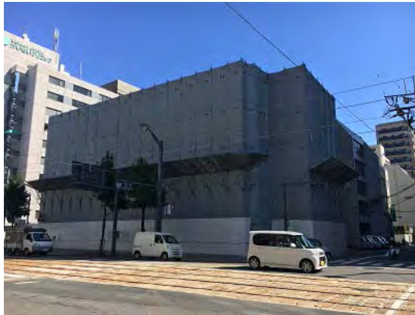
Existing building at the site which is currently undergoing demolition
