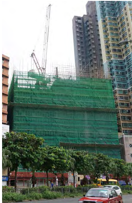
Site currently under construction
