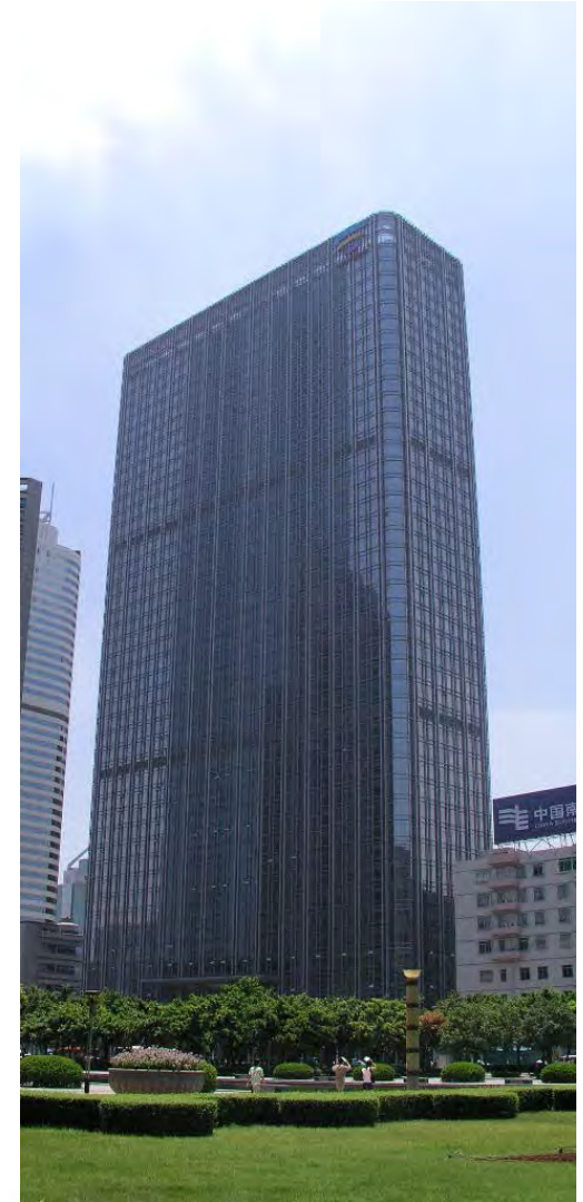
China Shine Plaza in Guangzhou, China
