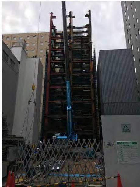
Current construction progress
