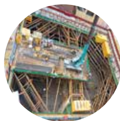
3. Site under construction
