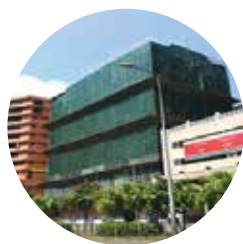
2. Original building while undergoing demolition
