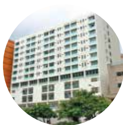
1. Original building on the land before demolition
